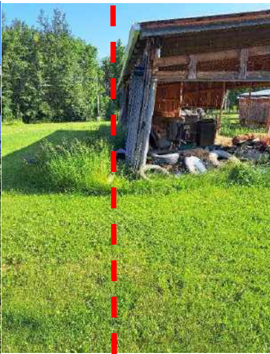
Illustration of the current lot line by the horse barn on lot 2.
