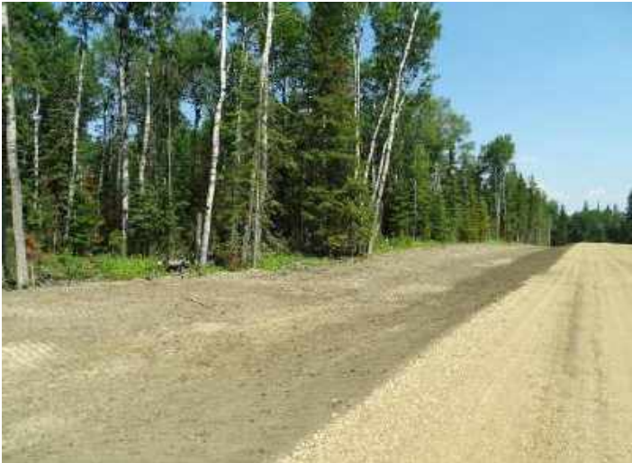
Drainage swale for the proposed road.
