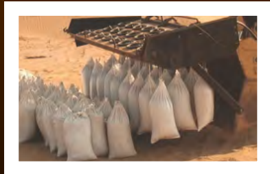
Placing the Sandbags
