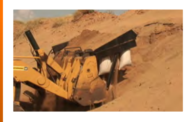
Transporting the Sandbags
